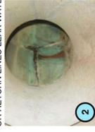
PROBLEM: CRACKS IN SUPPLY OR RETURN WATER SYSTEM UNDERMINES POOL BOTTOM AND CREATES CRACKS.
