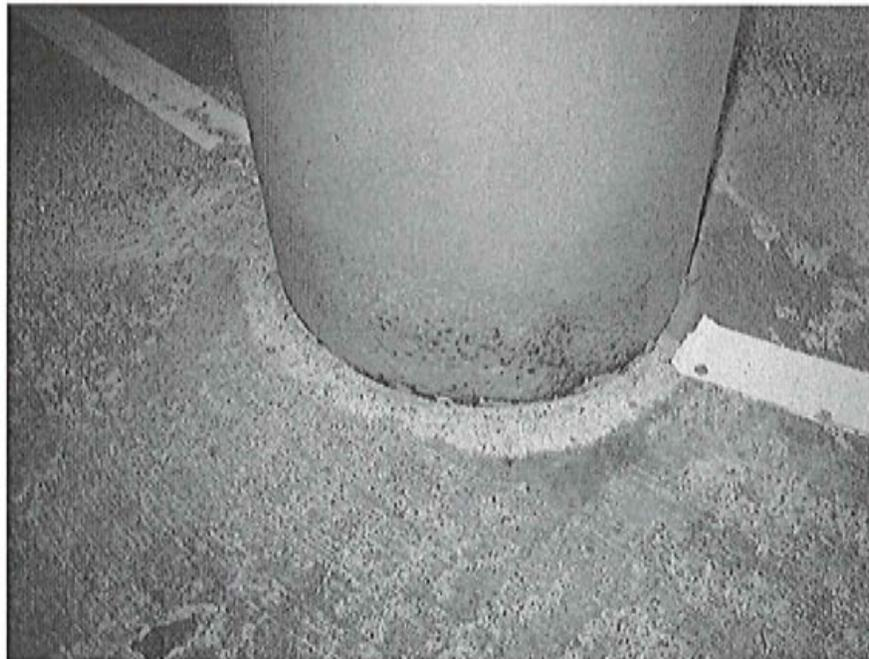
**(Photo #2) Typical sand blasted base of steel column pipe.**
