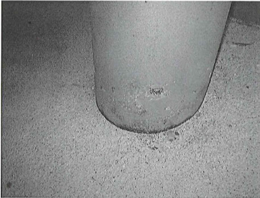
**(Photo #3) Typical sand blasted base of steel column pipe.**
