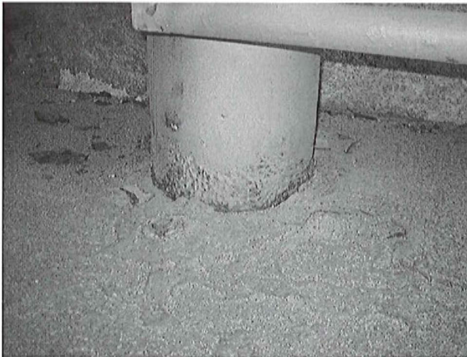
**(Photo #4) Slightly damaged steel pipe due to rust.**
