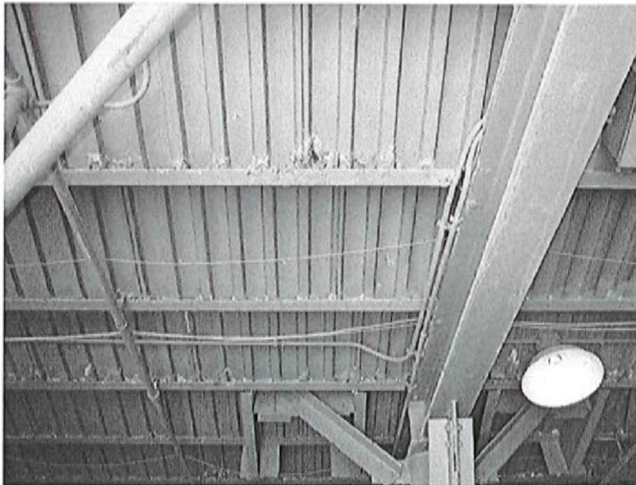
(Photo #9) Typical rusting on metal deck & channel beam.
