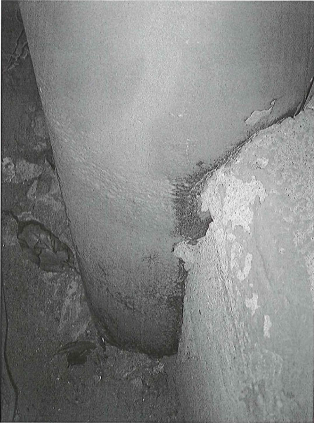
(Photo #5) Half of steel pipe column in contact with soil, dug, exposed & sand blasted.
