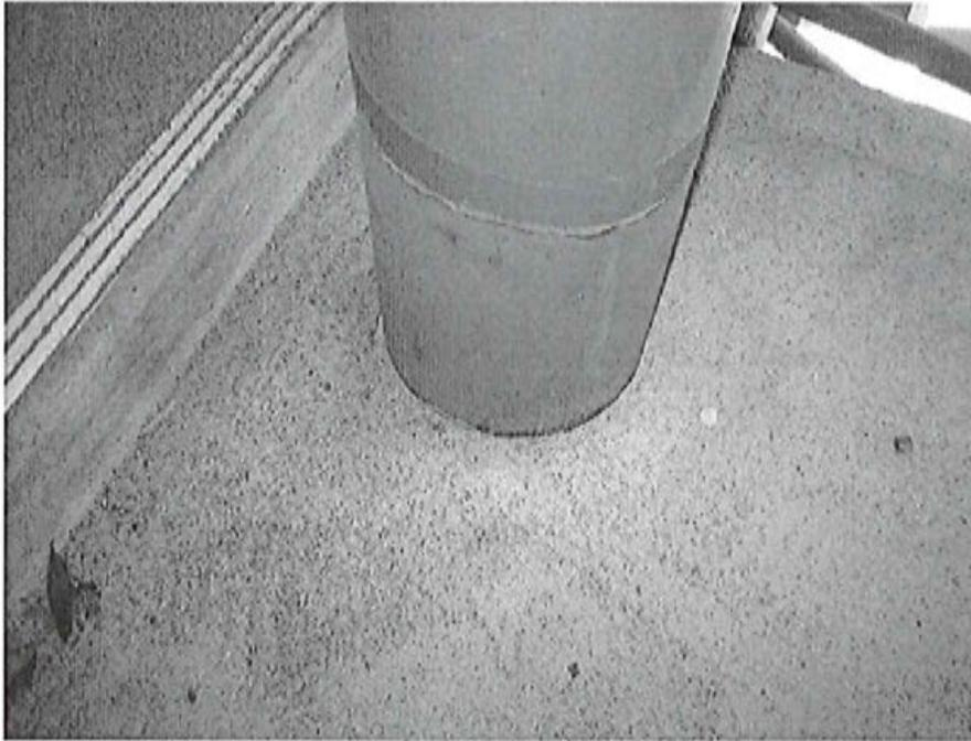
**(Photo #1) Typical sand blasted base of steel column pipe.**
