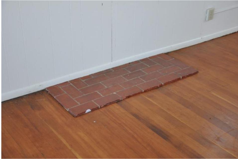
**Figure 41. U.S. Navy Radio Station & Barracks (#6), a brick hearth remains where the chimney was demolished. Source: Page & Turnbull, 2013**
