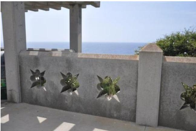
**Figure 76.** Detail of Park wall with star-shaped cut-outs and pyramidal-capped posts. Source: Page & Turnbull, 2014
