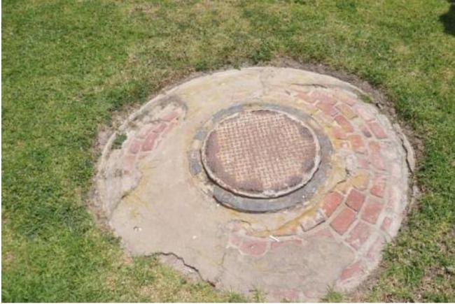
Figure 62. Brick and metal top of Cistern #14a. Source: Page & Turnbull, 2014
