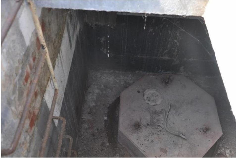
Figure 28. BES B'5 (#5) Interior with Octagonal Concrete Pad for DPF.
