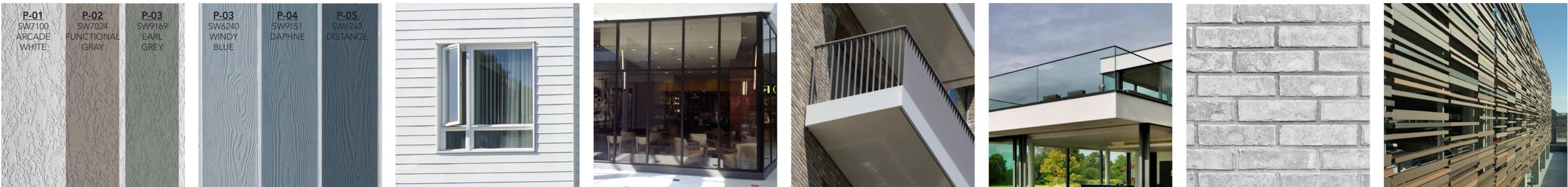
① CEMENT PLASTER      ② FIBER CEMENT SIDING      ③ VINYL WINDOW COLOR: WHITE      ④ ALUMINUM STOREFRONT NON-REFLECTIVE METAL      ⑤ METAL RAILING COLOR: SATIN BLACK      ⑥ GLASS RAILING NON-REFLECTIVE METAL      ⑦ MANUFACTURED BRICK COLOR: SW7100 ARCADE WHITE      ⑧ METAL GARAGE SCREEN FINISH: SATIN
