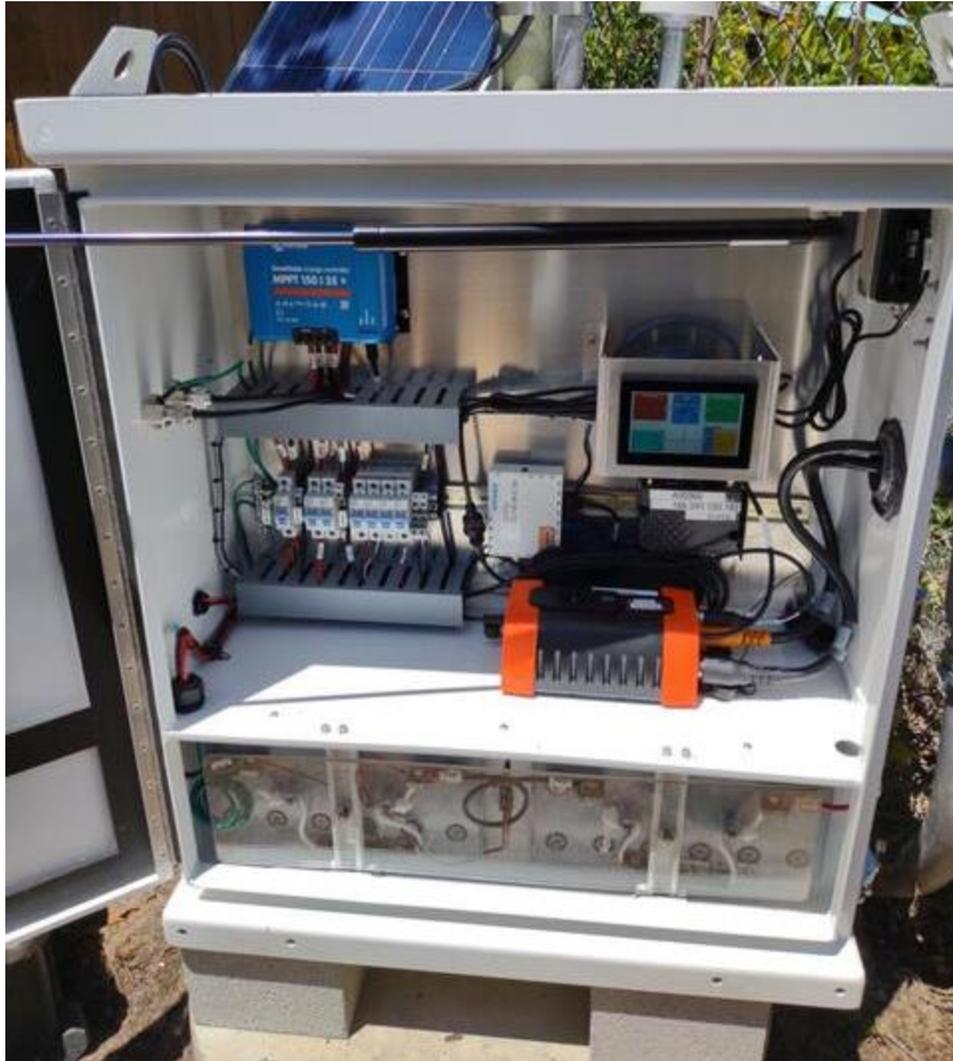
Example of similar cabinet, completed with electronics. Houses batteries, radios, charger, timing device, power controller. Everything will be grounded to a grounding rod.
