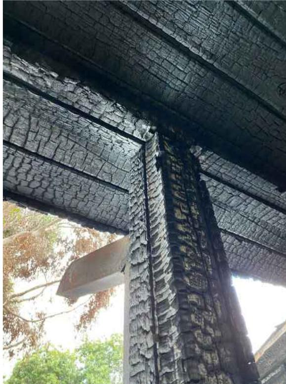
**Photo 26: Beam to Column Connection**
