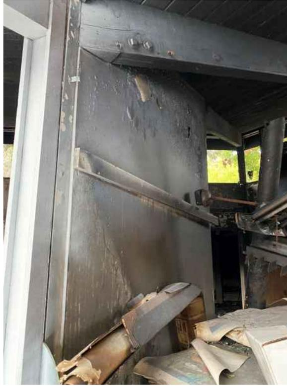
**Photo 38: Undamaged Bearing / Shear Wall**
