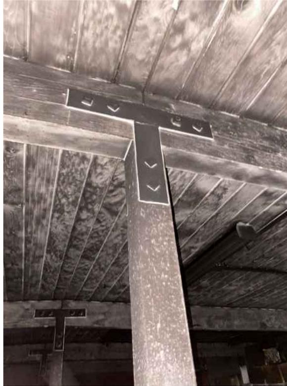
Photo 20: Typical Beam to Column Connection
