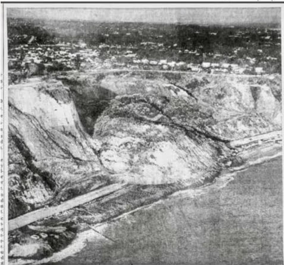
**JUTTING INTO OCEAN** off Pacific Coast highway between Santa Monica Canyon and Sunset boulevard are 600,000 tons of rain-loosened earth which took life of highway superintendent and upset heavy equipment. New cracks appeared in Via de las Olas on face of cliff after slide. All four lanes of usually heavily traveled highway are covered under about 100 feet of debris. (Roberts News Photo by Norman Wesler from Lind Flight Service plane piloted by Mel Lind.)
